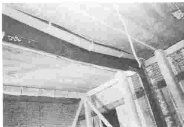
Figure 9. Condition of the test beam on completion of the fire test.
