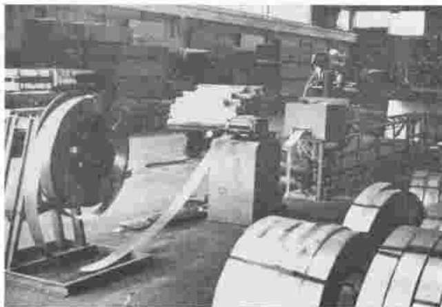
8 Colorcoat cut-up line (note plasterboard stacking area in background)
