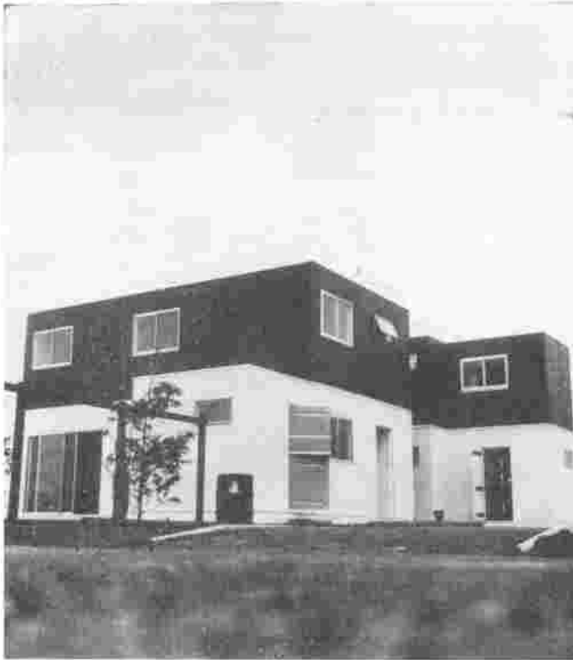
1 Two cluster-type IBIS prototype houses built to MOHLG Welsh Office requirements
