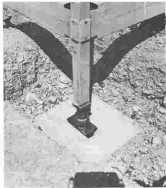
3 Adjustable column foot and precast foundation pad
