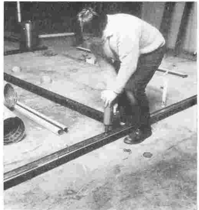
13 Partition track being shot-fired on to the floor screed
