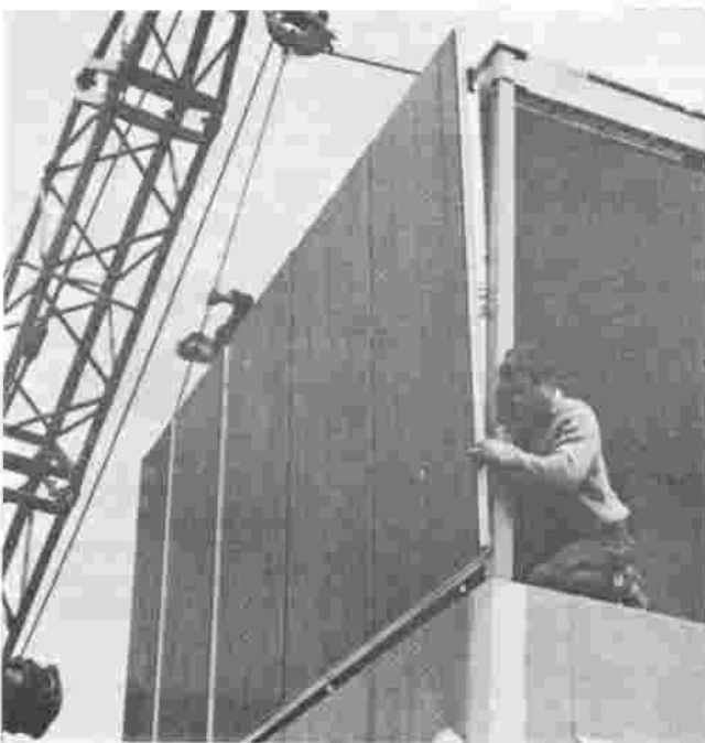
5 Erection of large wall panel at first-floor level
