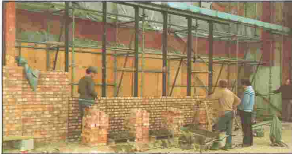
Figure 7 Masonry fire wall under construction showing embedded steel plates
