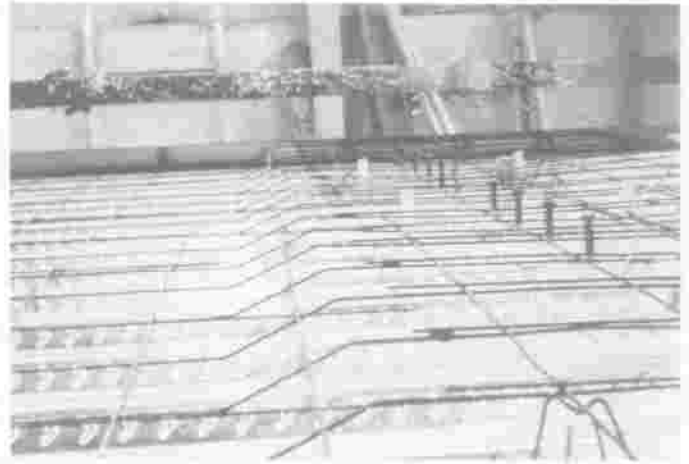
Fig 8. Cranked reinforcement used in FRS-BSC tests
