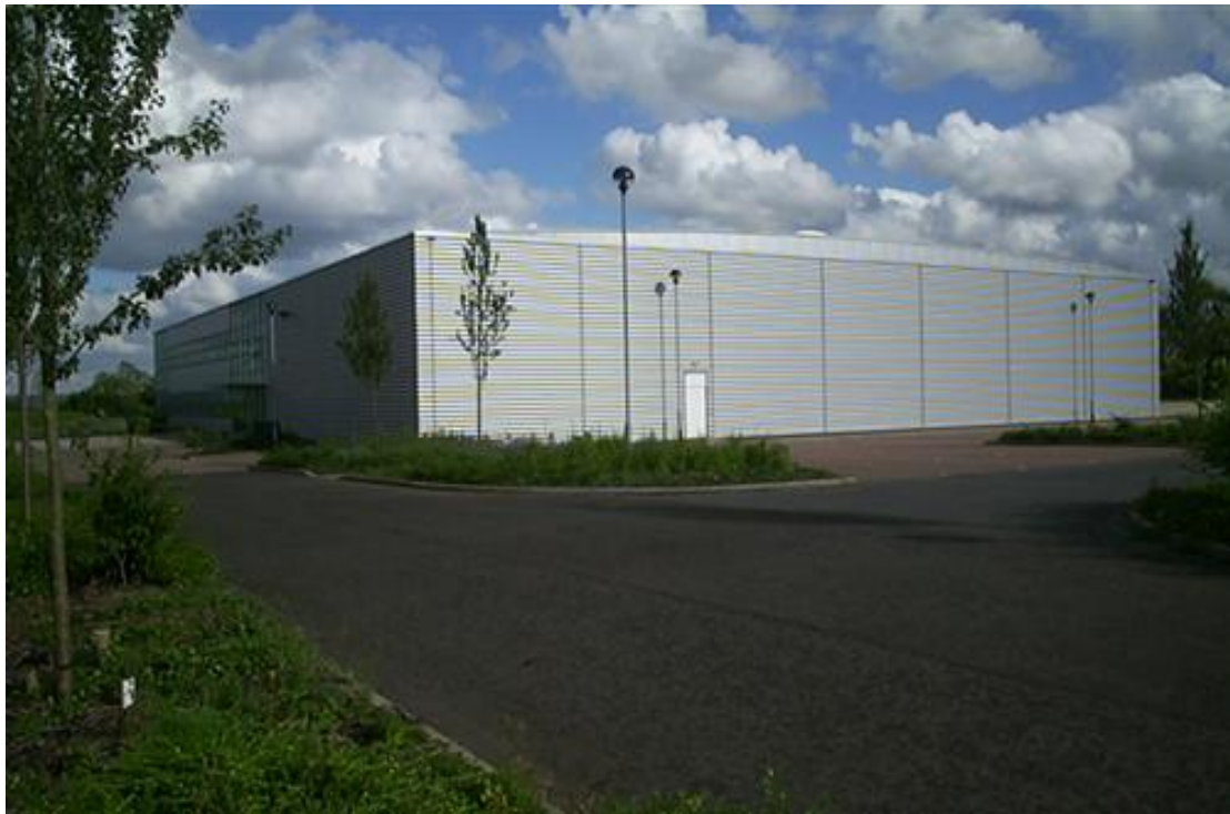
High Technology Units C, D & E, Phase 4 of Hamilton International Technology Park, Nr Glasgow.
