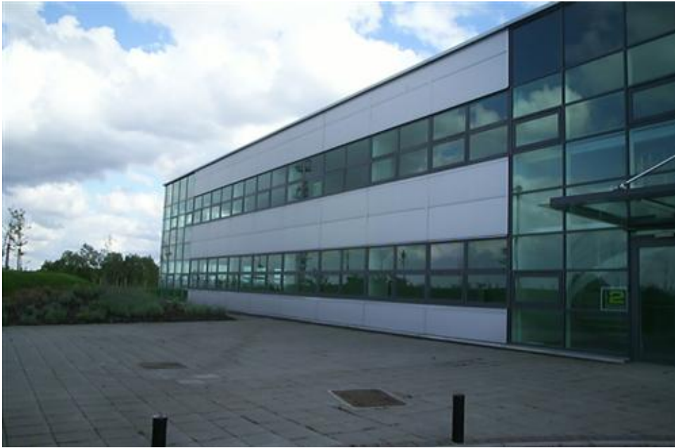
High Technology Units C, D & E, Phase 4 of Hamilton International Technology Park, Nr Glasgow
