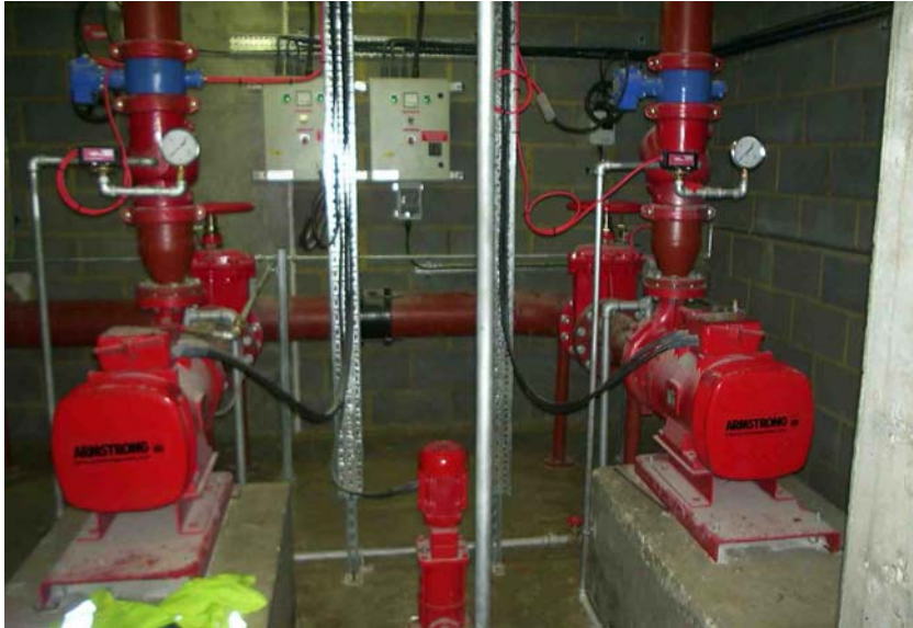
Life safety sprinkler pump installation in basement plant room.
