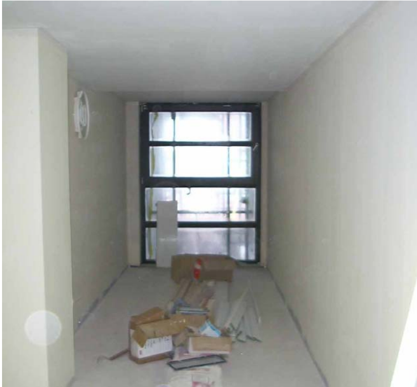
Cross-corridor smoke ventilating window in residential tower block during construction
