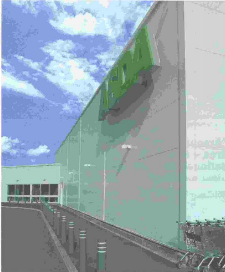
Rockspan panels used to provide a smooth appearance for an Asda superstore
