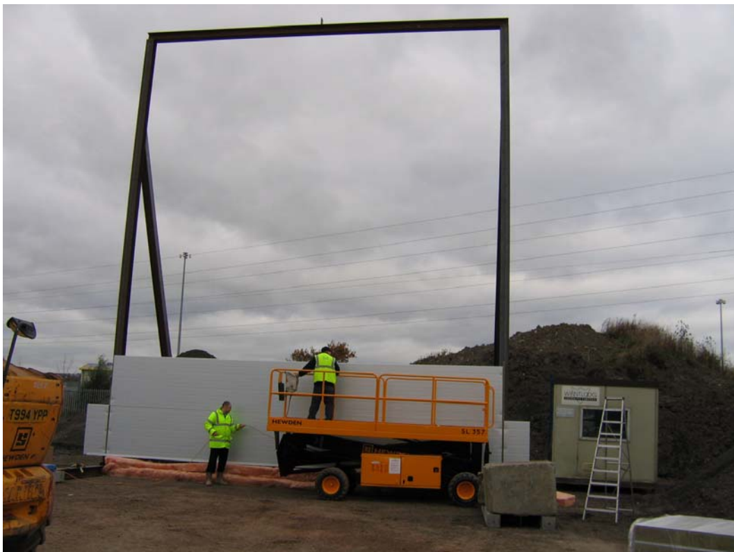
Steel frame with lower panels being erected
