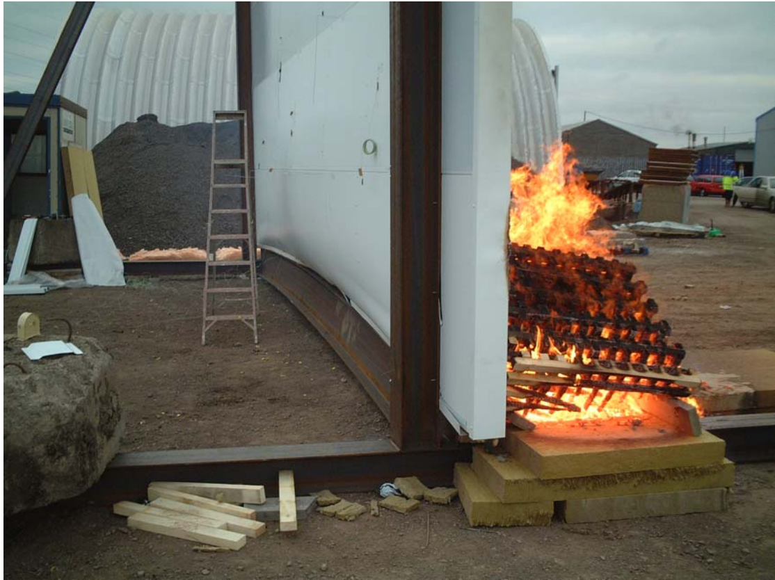
View along unexposed face toward end of severe fire test. Note good fire integrity of panel joints despite some bowing near the base.
